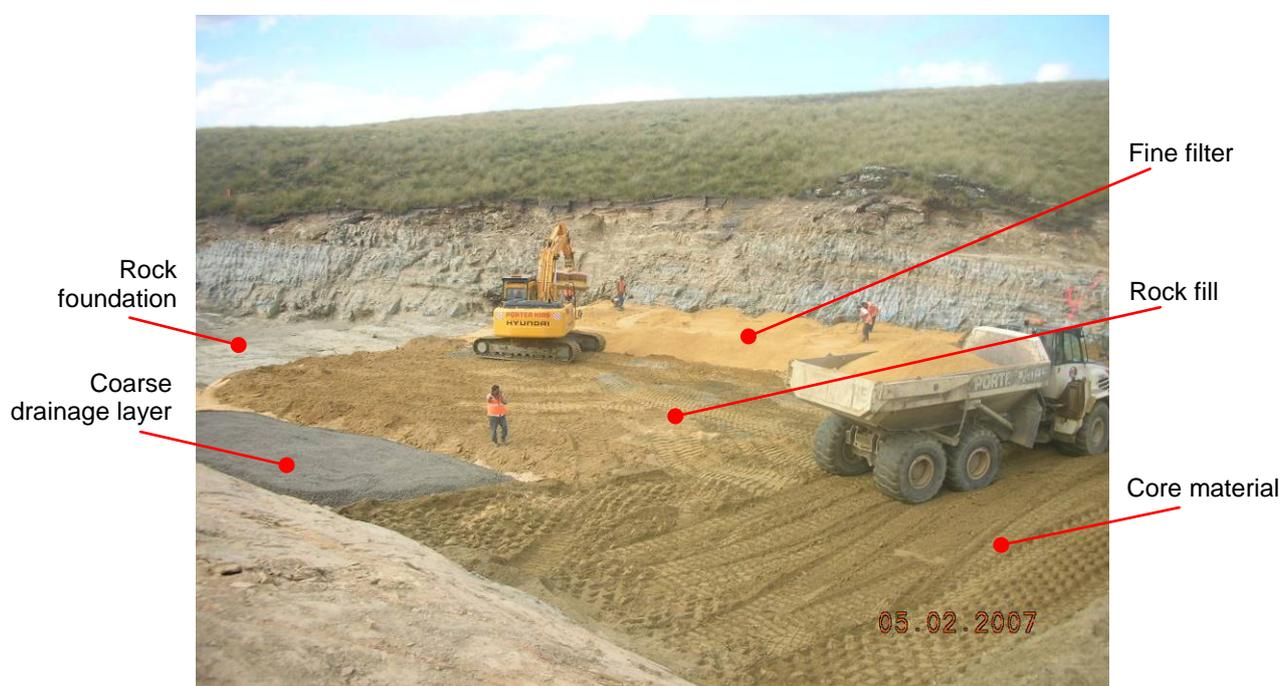
Photo 1: Main dam showing the dam core and the various drainage layers
