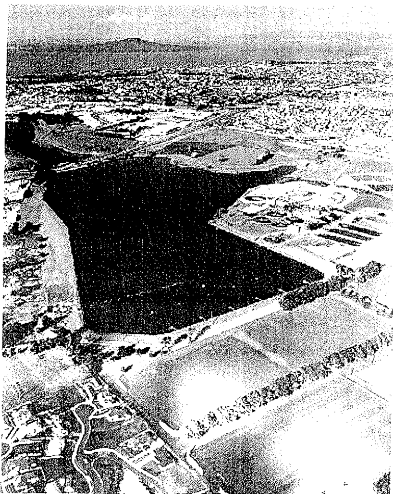
Figure 1. Rosedale Dam and North Shore City, with Rangitoto in the background.
