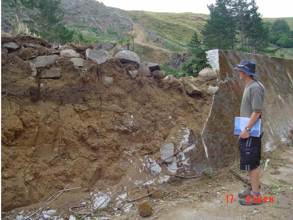
**Photo 1 : Demolition of the existing sidewalls**
